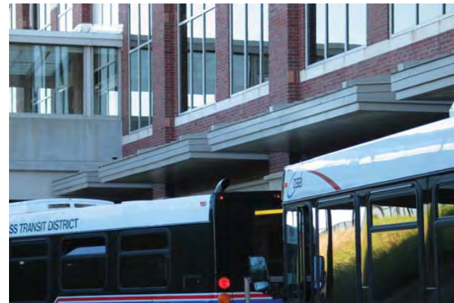
The Illinois Terminal, completed in 1998, serves as the center piece to the Champaign-Urbana Mass Transit District's city-wide bus service.
