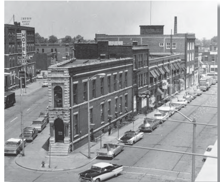
The Flat Iron Building, a landmark in downtown was demolished to create additional parking for Sears and Roebuck Co. in the mid 1970's. The effort was not enough to keep large department store anchors following the grand opening of Market Place Mall.
