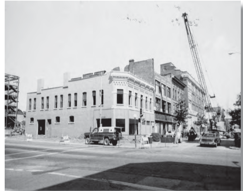
Nail Street and University Avenue looking northwest as demolition of the IOOF building proceeds.
