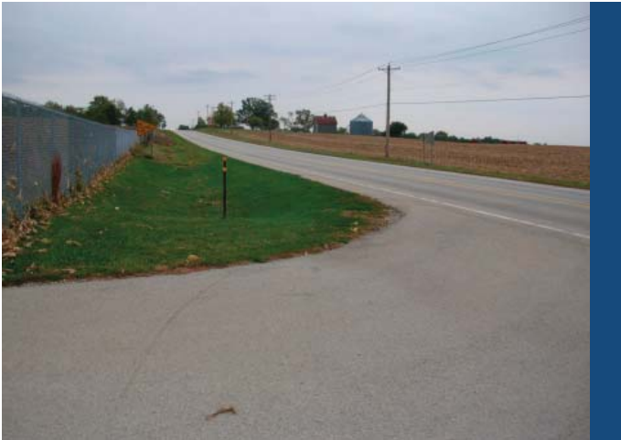
Entrance/exit to site looking east along Route 150.
