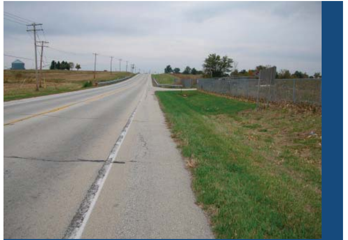
Entrance/exit to site looking west along Route 150.
