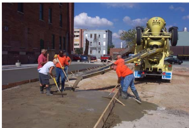
Pouring a portion of the parking lot near Carmen's Restaurant.
