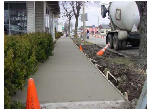
Newly poured sidewalk
