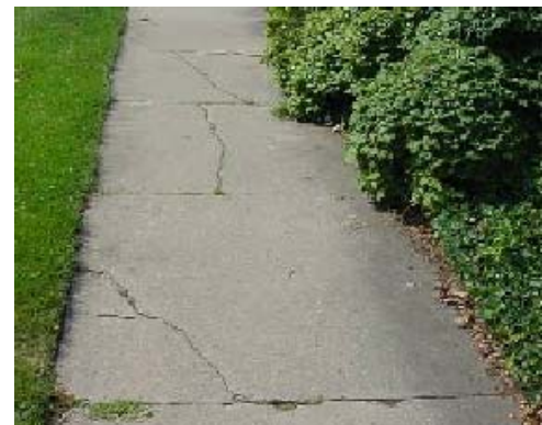
Broken Sidewalk (More than two pieces in one slab.)
