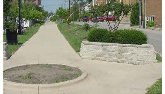
Sidewalk and retaining wall in the Boneyard area.
