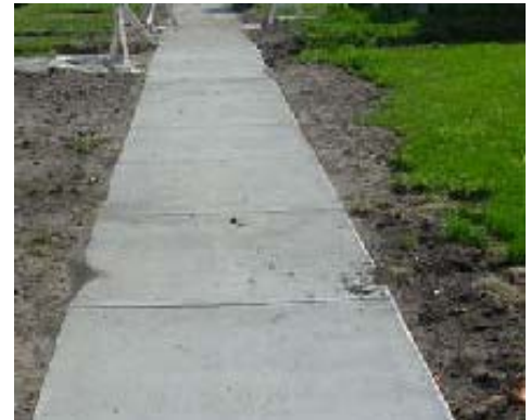
Soil restoration at a sidewalk repair location.
