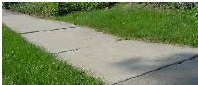
Settled, or sunken, sidewalk section.
