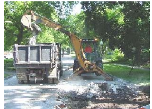
Sidewalk removal project.
