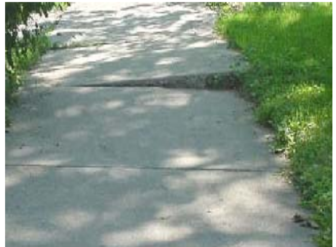
Buckled sidewalk (tripper).
