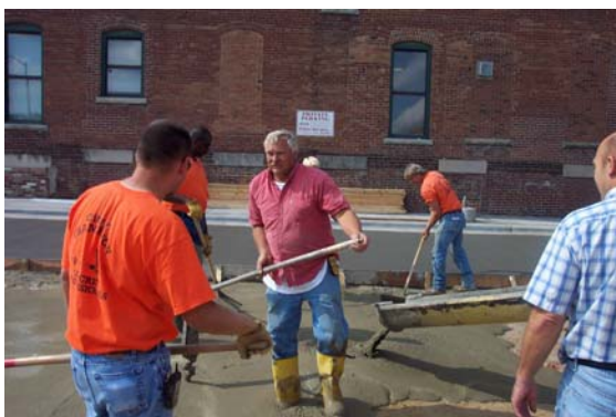
The Concrete Crew pouring the parking lot near Carmen's Restaurant in Downtown.
