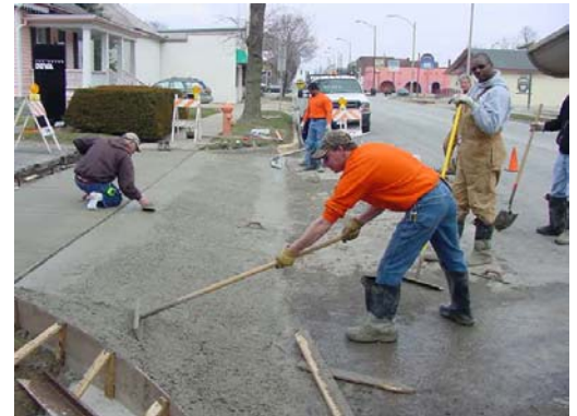
Concrete Crew repairing sidewalk and drive approach.
