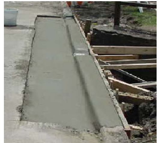
Box culvert repair.
