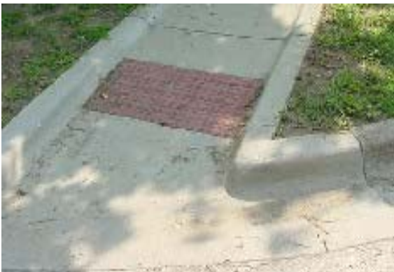
Single sidewalk access ramp.
