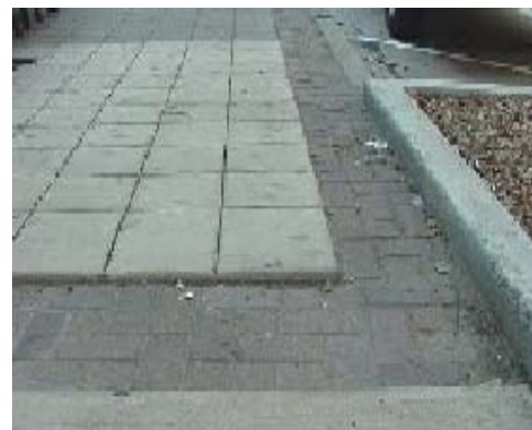
Possible trip hazard in a Streetscape area.
