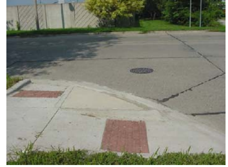
Sidewalk access ramps.
